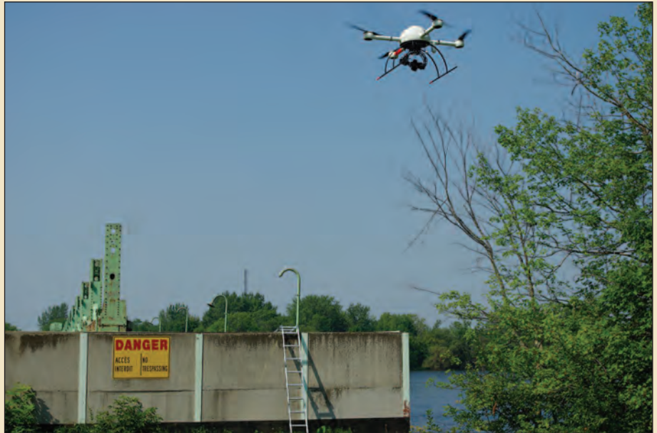
When dilapidated structures are too dangerous for human access, UASs provide a safe, cost-effective way to complete surveys and inspections.
