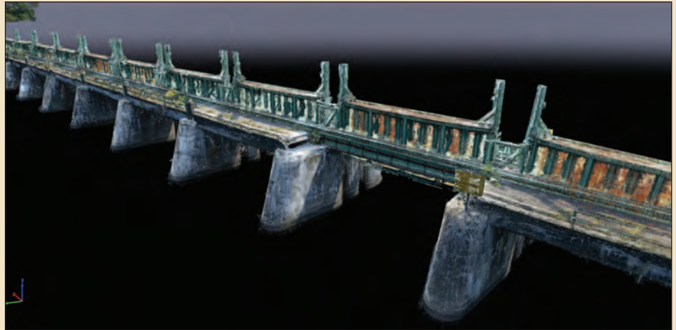
Using highly accurate data collected using a microdrones UAS, a preservation agency was able to create a 3-dimensional model of the dam that engineers could use when drafting their restoration proposals.
