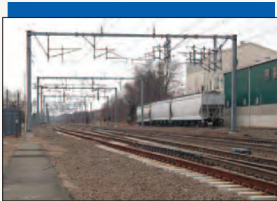
Example Electrified Railway
