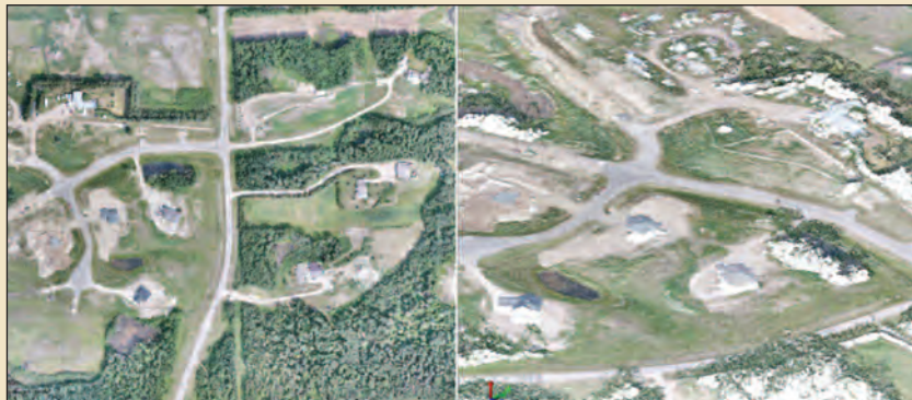
Figure 5: Point cloud (right) and orthomosaic (left) for the same area scanned in the earlier section
