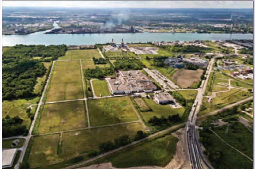
Gordie Howe International Bridge - Early Works September 2015. Credit: Front Page Media Group.
