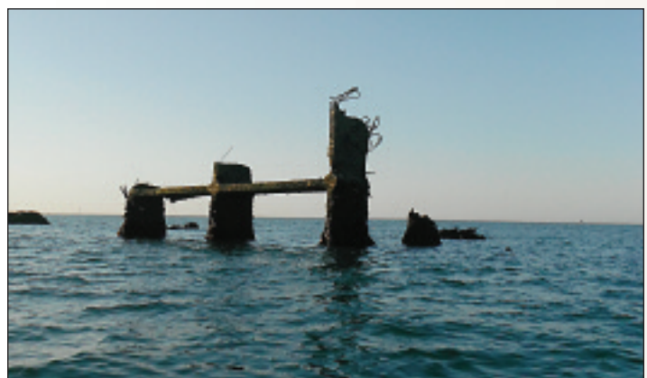
Some of the dangers that remained submerged at high tide but became exposed at low water. The vertical concrete structures and extruding rebar constituted a very real danger for the survey boat.
