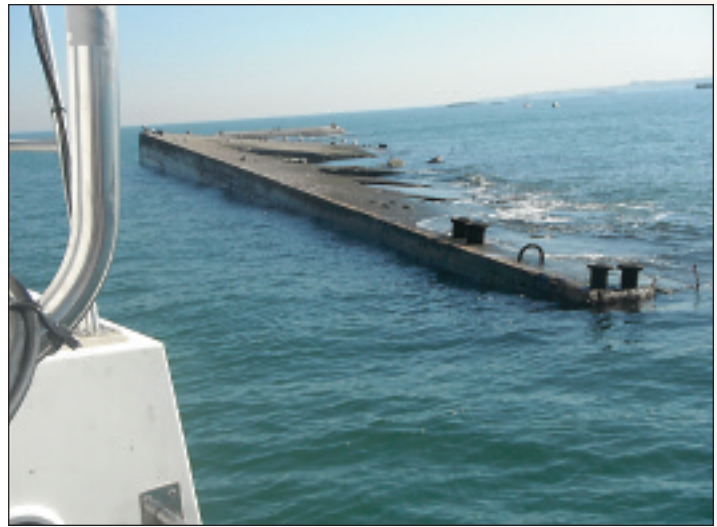
Navigating close to nearly submerged caissons at low water. These caissons are the large AX type, which are 200 feet long, 60 feet wide and 60 feet high. The boat is about 20 feet off the caisson. Only the extremely calm conditions allowed the boat to be this close.
