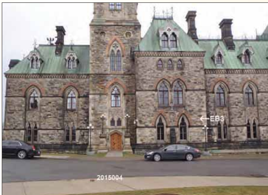
Figure 1: The control network is made up of monuments on the ground and prisms mounted on the walls of the buildings. Here, there are two points near the East Block. Some points, including 2015004, were installed to connect the existing interior networks of the Parliament Buildings to the new geodetic network.
