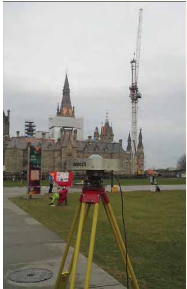
Figure 3: GNSS survey session at point PPD2015 H20 in front of the West Block construction site.
