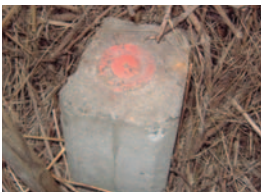
MTO Concrete monument
